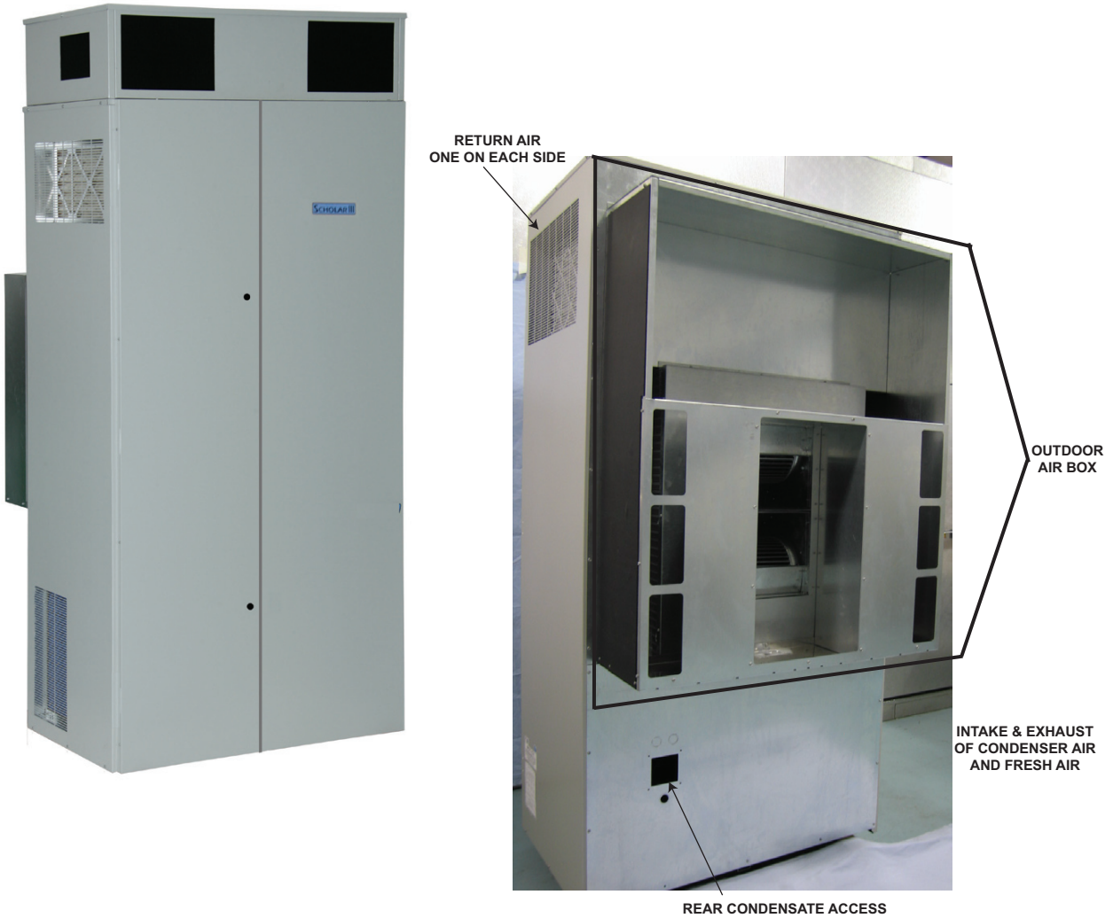
Figure 1. General External Component Identification and Access to Scholar III™ Heat Pump or Air Conditioner
